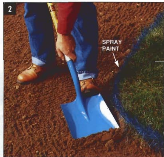
REMOVE SOD in an area extending 8 in. beyond the boundaries of the patio. Spray paint indicates the excavation line.
